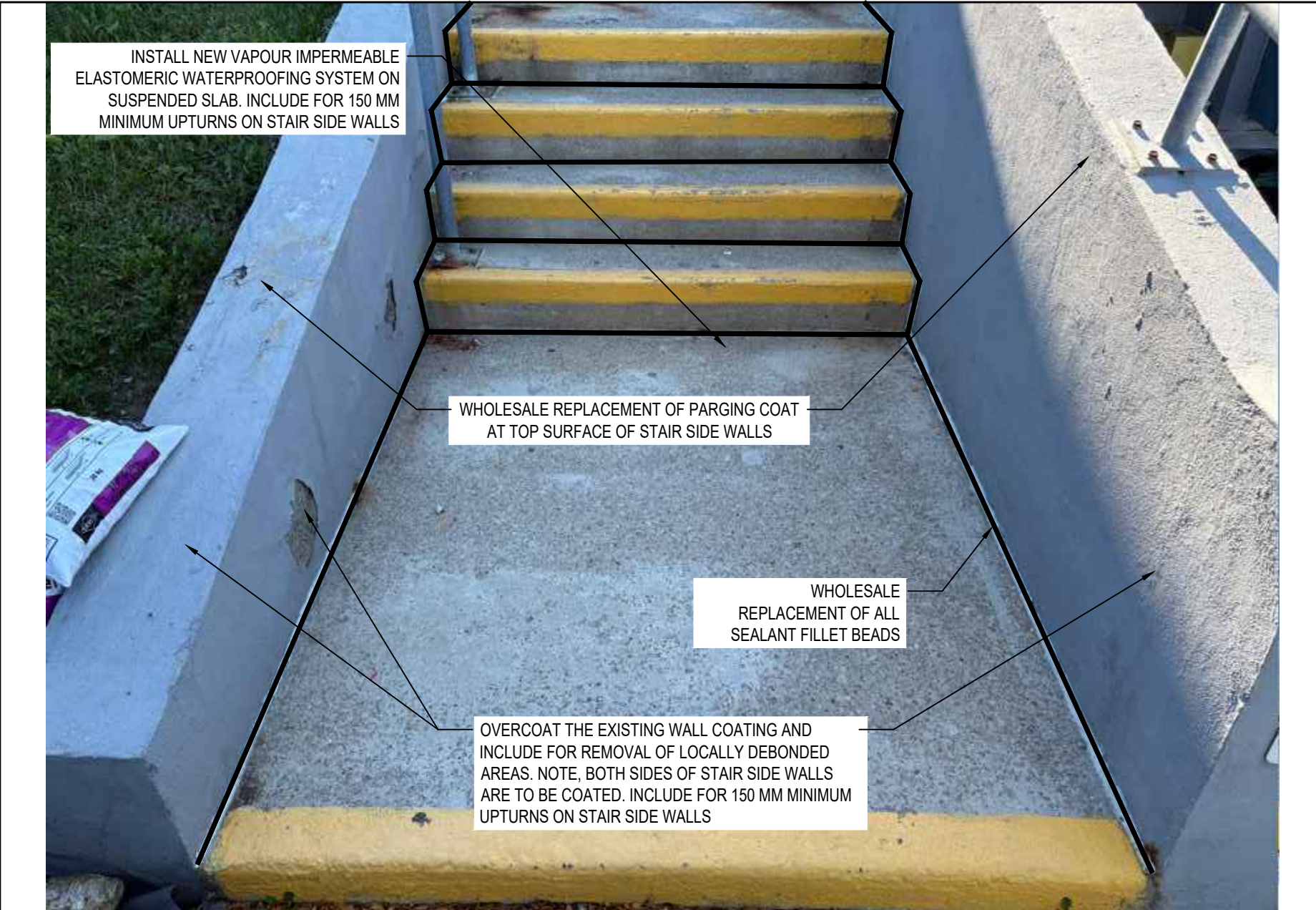
3 TYPICAL VIEW OF SUSPENDED STAIRS AT NORTH WEST LOADING DOCK SCALE: NTS
